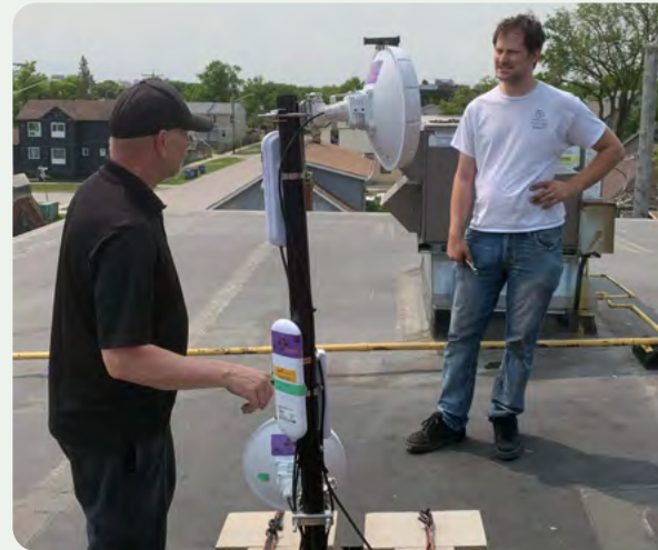
Installing antennas in Winnipeg’s North End. © Internet Society Canada Manitoba Chapter.
