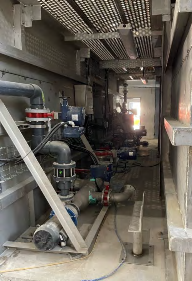
Water Filtration Plant Construction Progress
